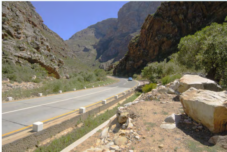
Road and Pavement Rehabilitation and Maintenance
