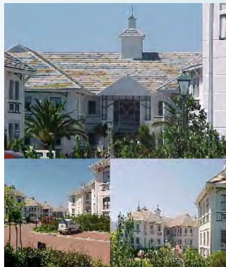
AINTREE OFFICE PARK R 25 million
