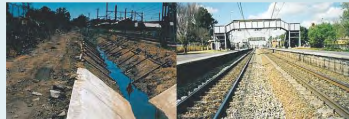
METRO STATIONS PERWAY DRAINAGE & SLOPE STABILITY R 64 million
