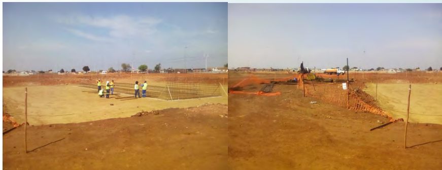
KATLEHONG LICENCING HUB BULK EARTHWORKS & STRUCTURES R 68 million
