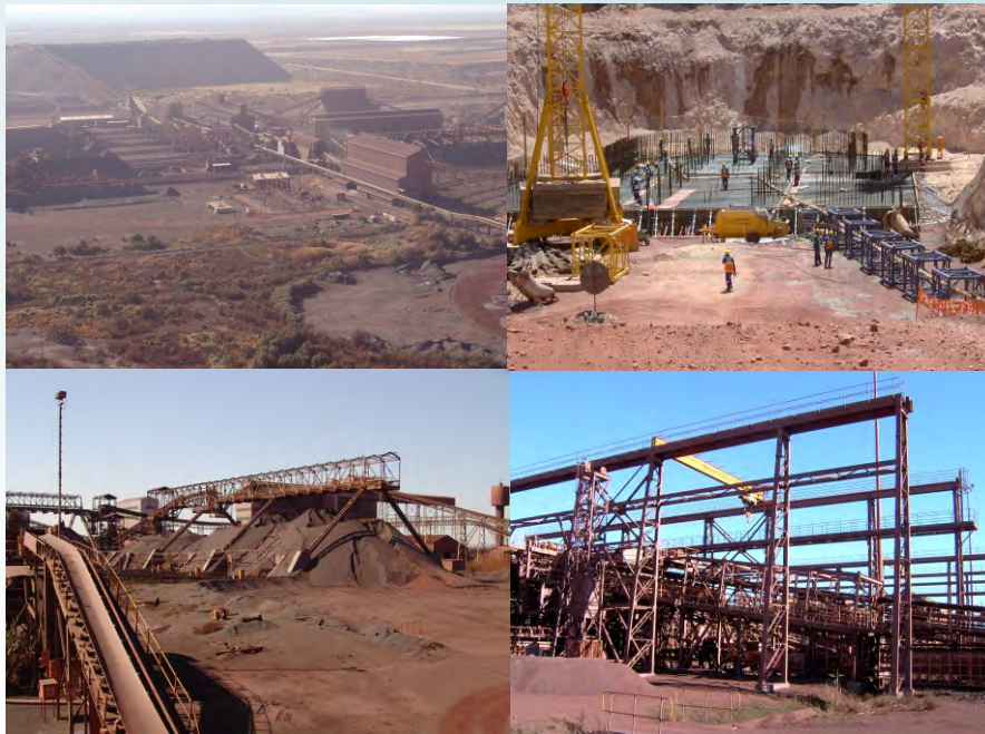
KUMBA IRON-ORE MINE R 350 million
