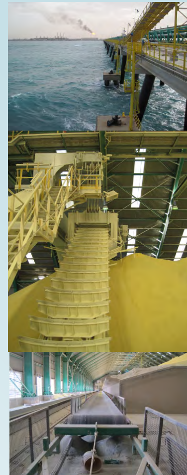
LIBYA SULPHUR EXPORT FACILITY REFURBISHMENT R 50 million
