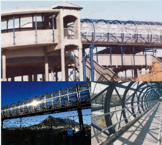
METRORAIL ACCESS BRIDGE R 15 million
